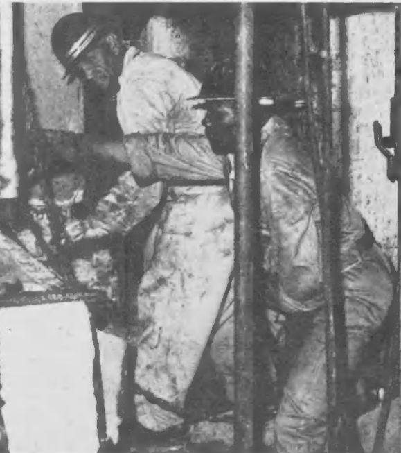
RIGGERS USE a chain block to remove a three-ton chunk of steel from the foundation of No. 5 Combination Unit, left. A hole is cut, center, to aid in rigging a block and tackle assembly. Nasario Tromp, metal trades foreman, right, inspects progress of the dismantling.
